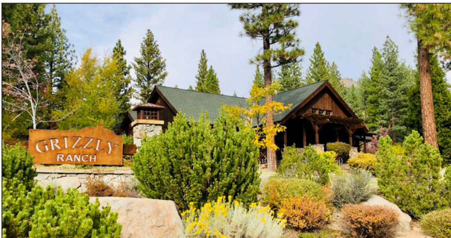
Wastewater problems at Grizzly Ranch included failing grinder pumps and a treatment system that was unable to handle the low flows that are common in the winter. (Photo courtesy of Pace Supply.)
