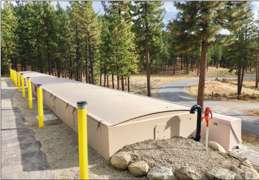
These two AX-Max™ units make up the Grizzly Ranch phase-1 installation, capable of treating up to 25,000 gallons (95 m³) per day. More units can easily be added as the development builds out. (Photo courtesy of Pace Supply.)
